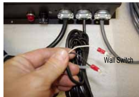
Figure 11. (Remote Switch Wire connection)
